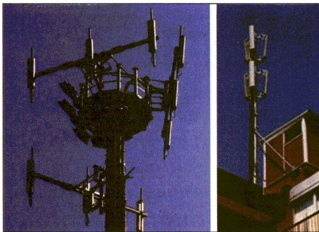
2. In a typical antenna system for a clover BTS for GSM (left), a common pole hosts the antennas for three adjacent 120-deg. sectors. A low-environmental-impact antenna is shown (right) for contrast.
